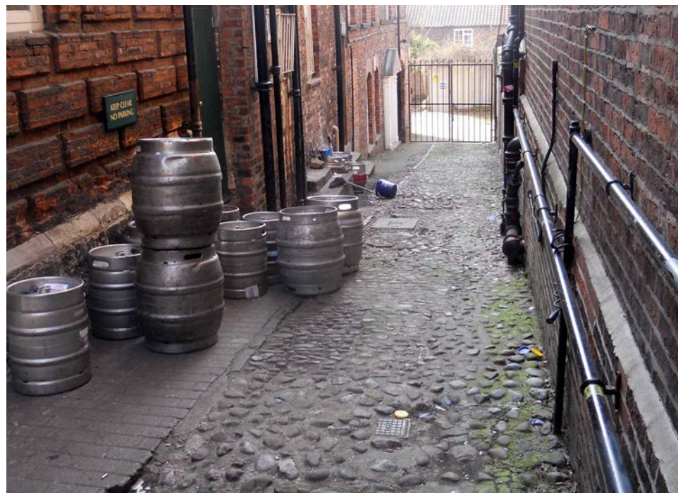
Private access lane to the River Ouse, off Lendal, publicly visible, adding richness to the character of York. The historic cobbles are however, poorly maintained and at risk. The clutter, sometimes including waste bins is a detractor.
