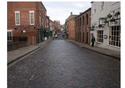
Dark granite setts on Foss Gate
