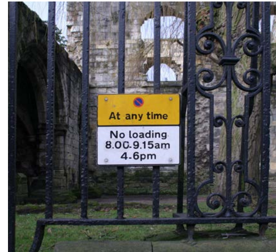
Sign fixed to listed railings detracting from historic setting and impacting on the railings.
