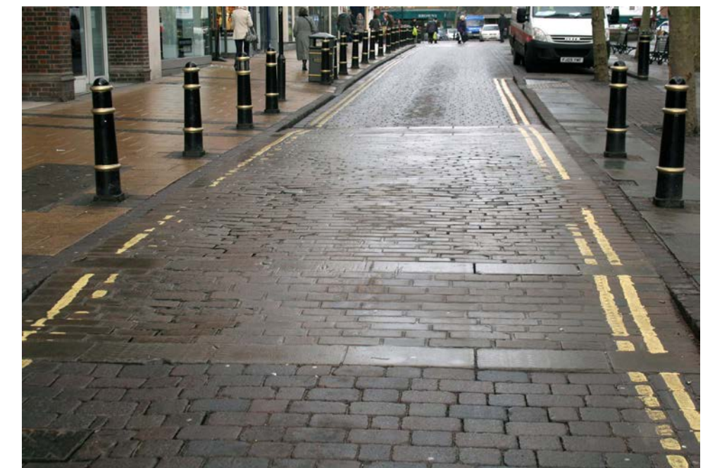
A well constructed raised table on Parliament Street consisting of English Pennine sandstone setts with pre-cast brick paviours on either side, providing level access across the carriageway.
