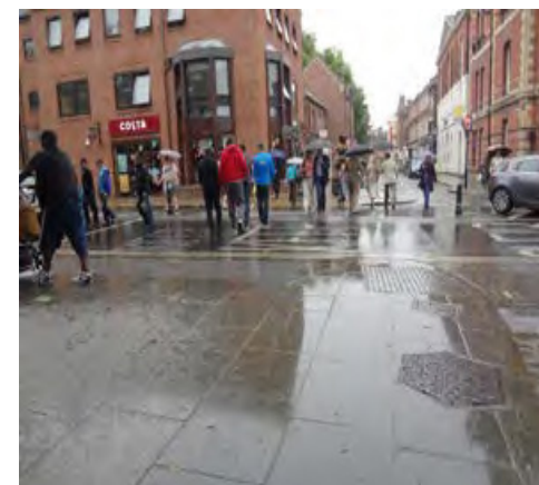
A very good example of a crossing with English Pennine sandstone blister paving on Museum Street
