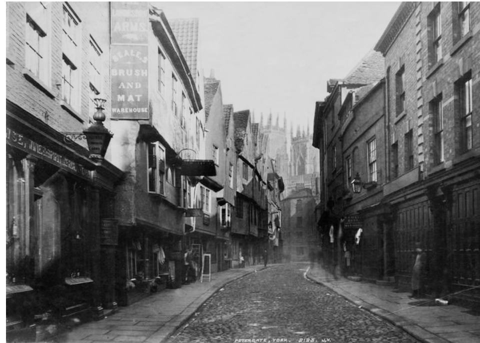
This 1880s photograph of Low Petergate shows the relationship between flagstone pavements, a good wide stone kerb and the carriageway with stone setts - all locally sourced English Pennine sandstone. (City of York Archives)
