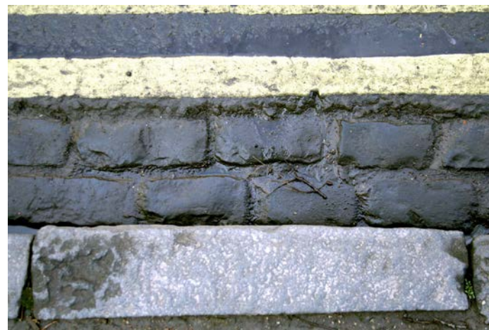
Traditional brick drainage channel in situ parallel to a granite kerb adding interest to the carriageway.
