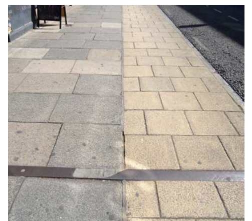
Two different materials used on Micklegate when the pavement was widened, resulting in an unattractive and uncoordinated footway
