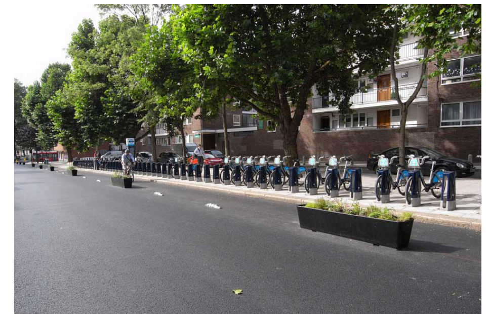
Planters used to demarcate a cycle track on Royal College Street, London
