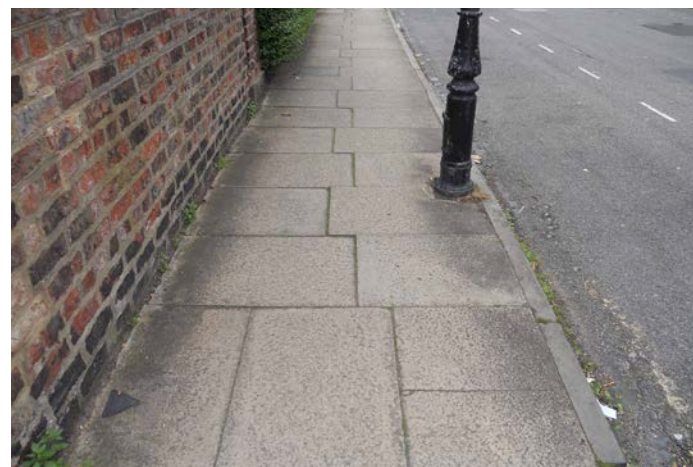
Although replacing traditional riven Sandstone flags, these staggered 1950s concrete paving slabs in Bishophill are more preferable to contemporary smaller pre-cast paving.
