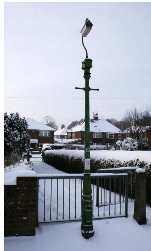
Street light from the 1950s with an attractive traditional swan neck fitting on Finsbury Avenue, off Bishopthorpe Road.
