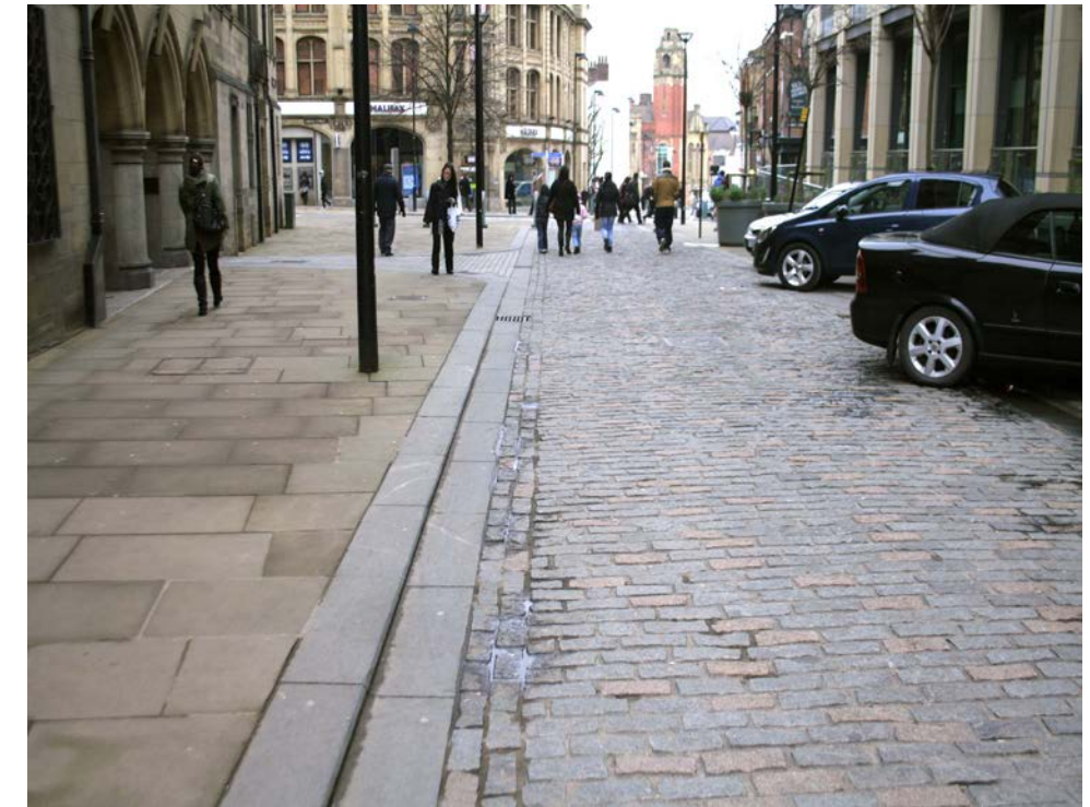
Good simple design in Sheffield using a small pallet of natural stone materials, in this case, granite setts on the carriageway, wide top granite kerbs and Marshall's Cromwell sandstone flags.
