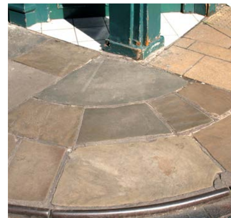
Well thought out approach to laying riven flags at a corner - note the original cast iron kerb, used to protect the pavement edge
