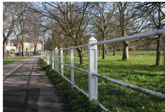
Unlisted railings at the Knavesmire
