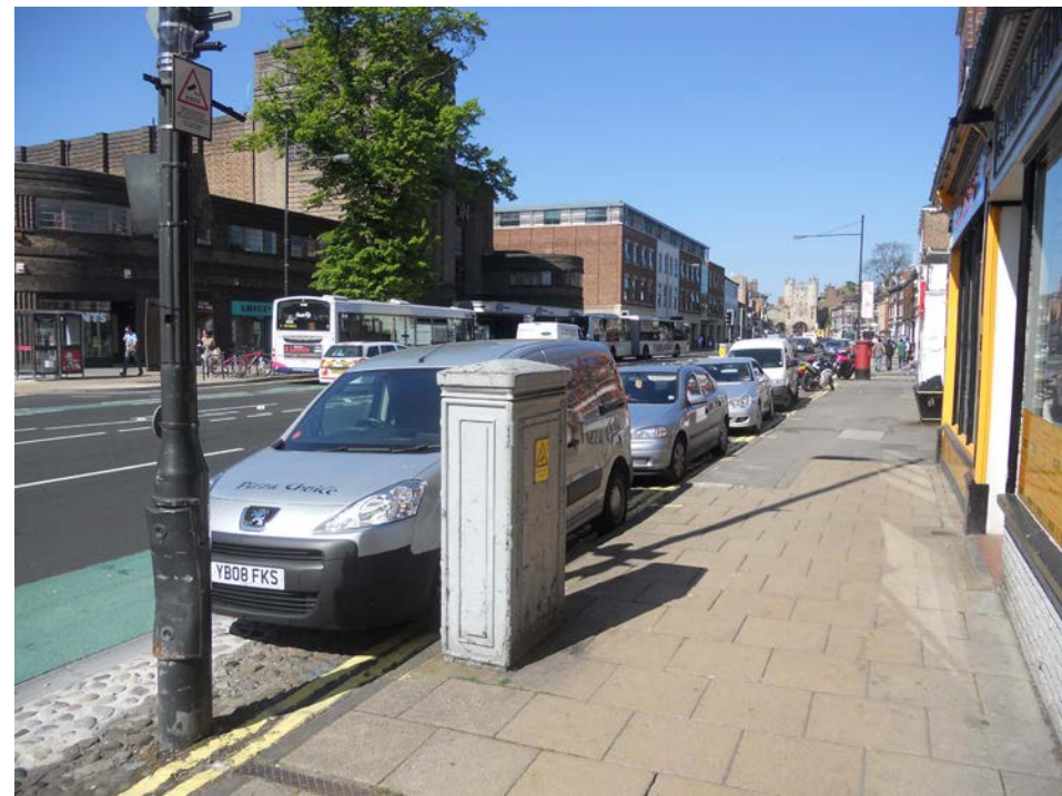
Blossom Street - recently improved through the re-modelling of several pedestrian crossings, improved cycle lanes and the removal of some signage. However, the gateway street contains several types of light column and street furniture is inconsistent. Repair and maintenance of surfaces is also inconsistent and sometimes poor quality.
