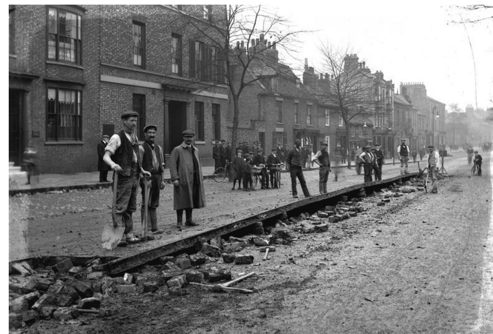
This photograph records a pause in electric tram track laying on Blossom Street in 1910, clearly showing stone setts, later replaced. (City of York Archives)
