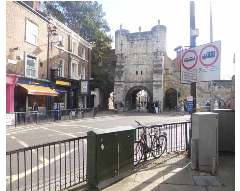
Railings at Bootham Bar - poor quality and combining with too many utility boxes significantly impacting on the setting of this important gateway into the city
