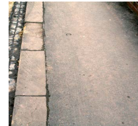
Tarmac pavement surface used to good effect with broad-top English Pennine sandstone kerb
