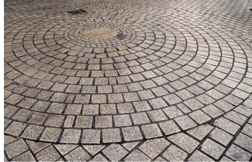
A fine example of the decorative use of blanc-de-bierge setts in Spurriergate
